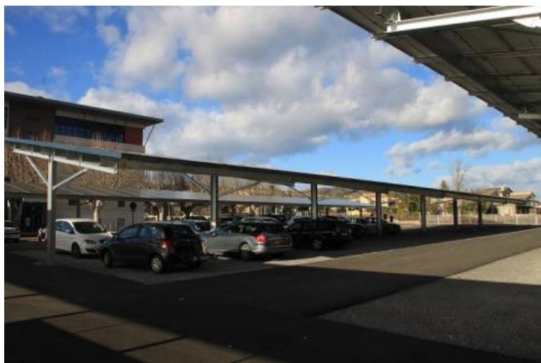
Parking gare routière
